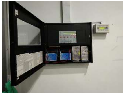
Main Control Fire Alarm (MCFA)
