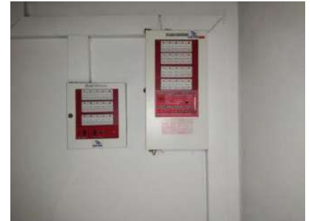
Main Control Fire Alarm (MCFA)
