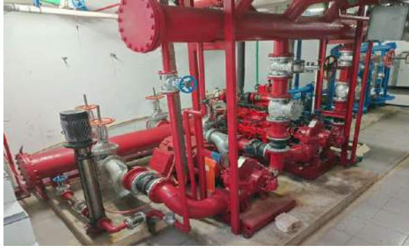
Pompa Hydrant
